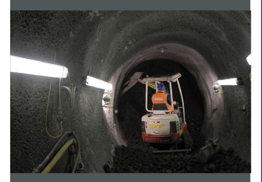
Works were to construct a new cable tunnel and shaft and tie into the existing Liverpool St underground station.
